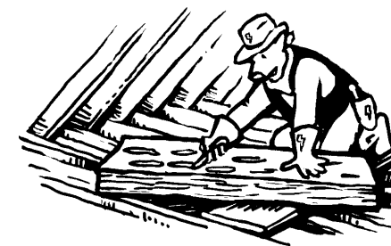
IF YOU INSTALL ADDITIONAL INSULATION, IT SHOULD BE UNFACED—OR USE A KNIFE TO FREELY SLASH THE VAPOR-BARRIER TYPE
