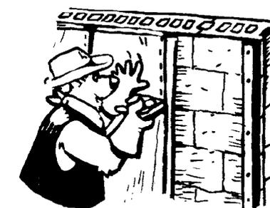
**INTERIOR BASEMENT WALLS CAN BE FURRED OUT WITH 2x4 STUDS AND INSULATED WITH GLASS FIBER, OR THE SPACE CAN BE FILLED WITH EXTRUDED POLYSTYRENE.**
