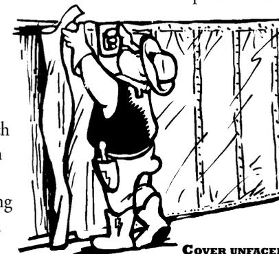
**COVER UNFACED INSULATION WITH A VAPOR BARRIER SUCH AS POLYETHYLENE PLASTIC.**
